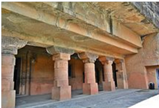
Cave 24; the Ajanta Caves were carved into a massive rock on the Deccan plateau
